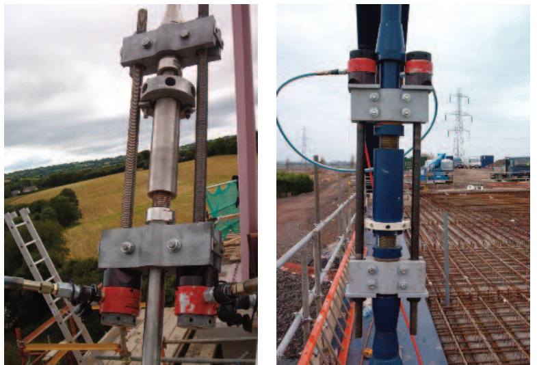
Daver Steels jacking frame on location
