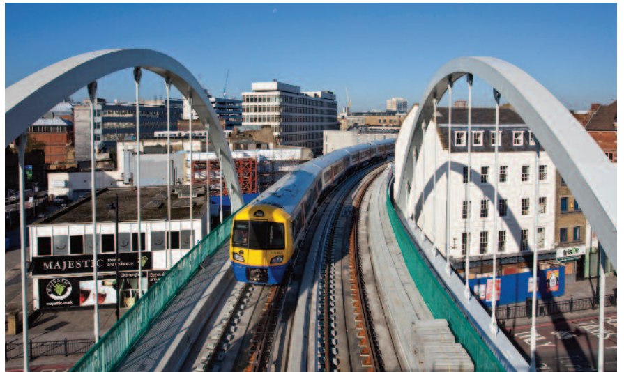
Shoreditch Bridge, London
